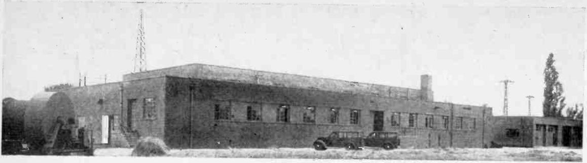
Post Office S-W transmitter station building at Criggion near Shrewsbury.
